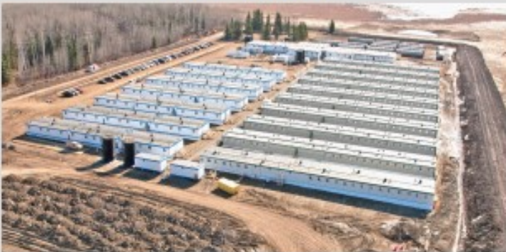
800-person work camp on Coastal GasLink pipeline
